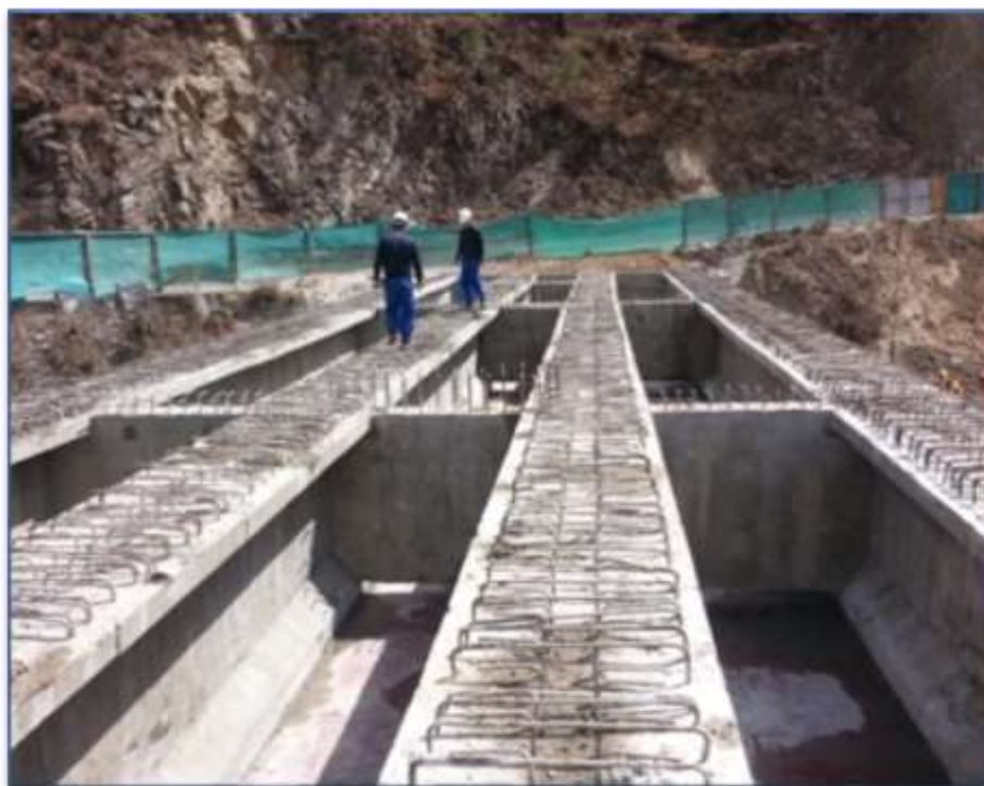
Figure 14: Casting of longitudinal girder and cross girder
