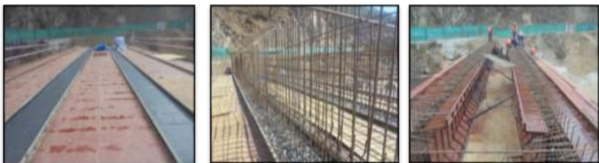
Figure 13: Fixing of platform, reinforcement bar and shutter for longitudinal girder casting
