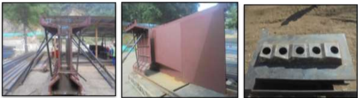
Figure 12: Fabrication of shutter for longitudinal girder (mid-section, transit and end shutter)
