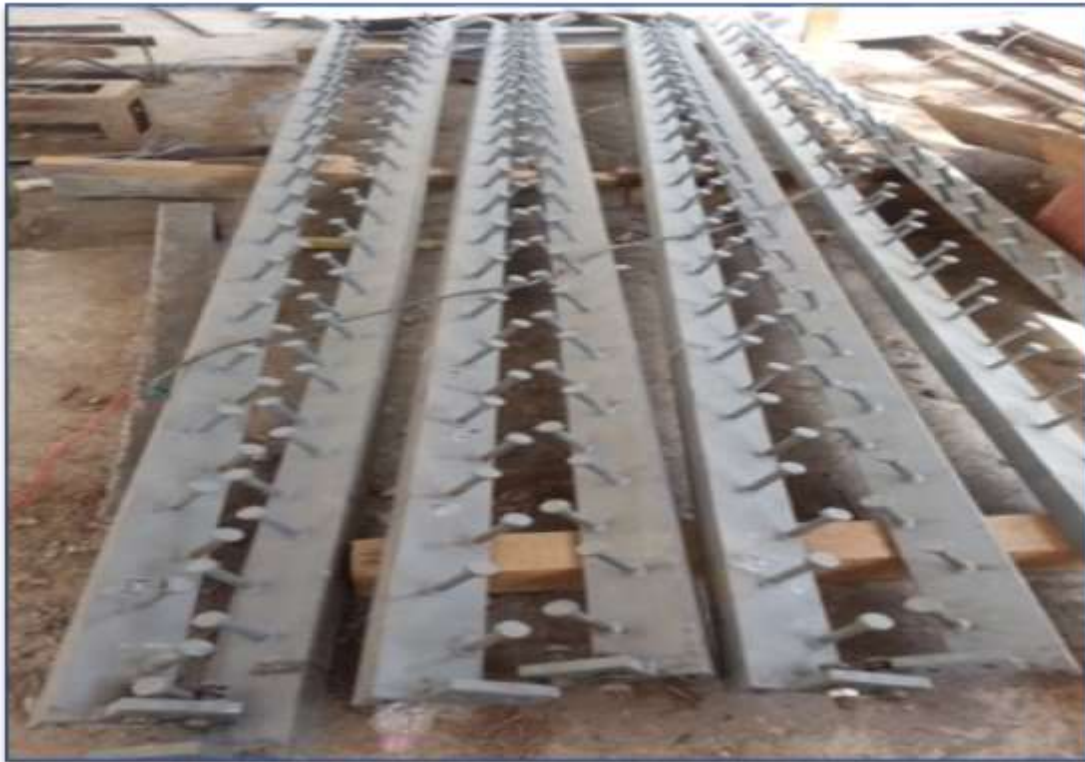
Figure 18: Strip seal expansion joint.
