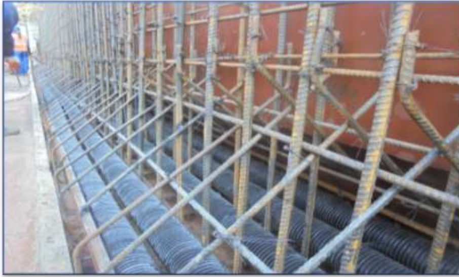
Figure 15: Tendon layout profile in longitudinal girder
