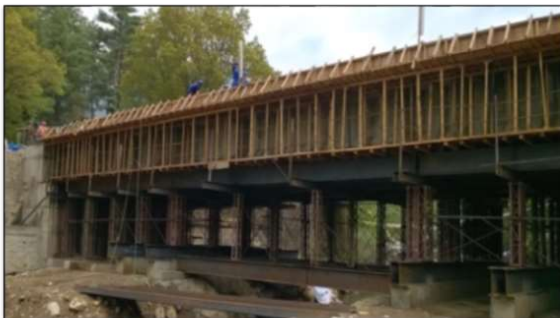
Figure 10: Staging for construction of superstructure
