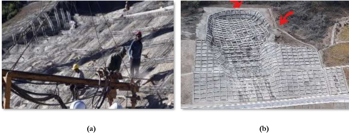
Figure 7. (a) Drilling being done for installation of subsurface drainage; (b) Completion of installation of drain pipes for subsurface, periphery drainage gutter and completion of shotcrete work
