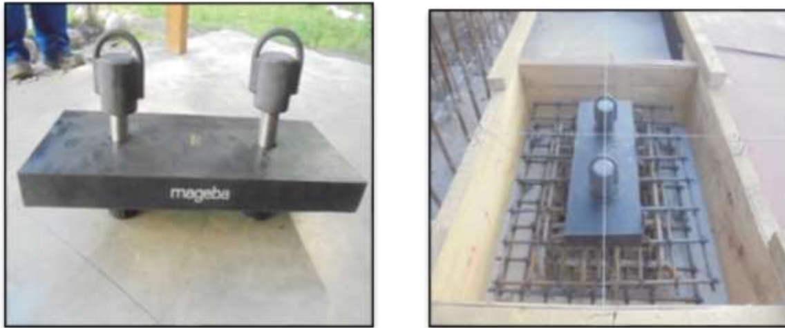
Figure 11: Bearing placement on abutment
