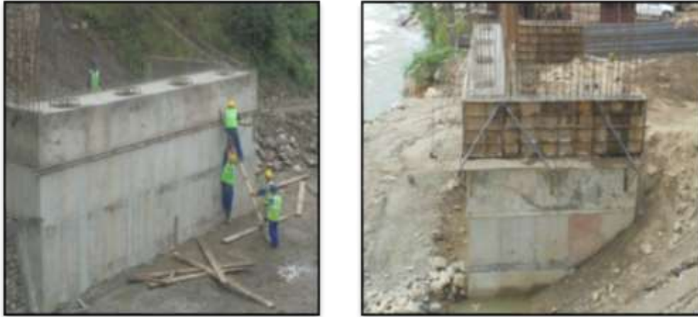
Figure 9: Construction of Abutments
